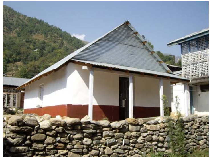
Jabori Straw Bale Women's Community Center, 2006
